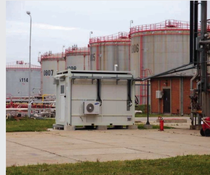
Analyzer house for process analytic in Refinery Pančevo with 12 analyzers for optimisation combustion process in furnace
