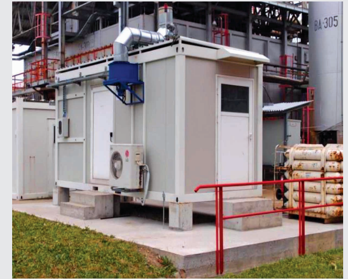
Analyzer house for measuring quality fuel in Refinery Pančevo Designed for installation in the Ex zone
