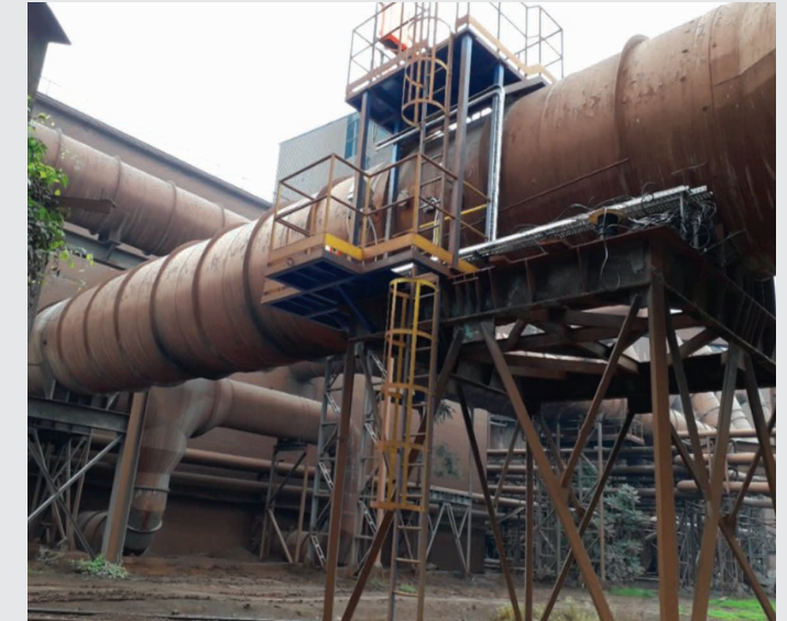
Access platform for measuring equipment on channel the steelworks in the HBIS-Smederevo
